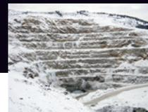
**Our 2007 geotechnical study recommended a 5° increase** to the pit slopes of Capstone's Minto copper-gold mine in the Yukon. Estimates suggested this would reduce waste stripping by ~4.5 million tonnes.
